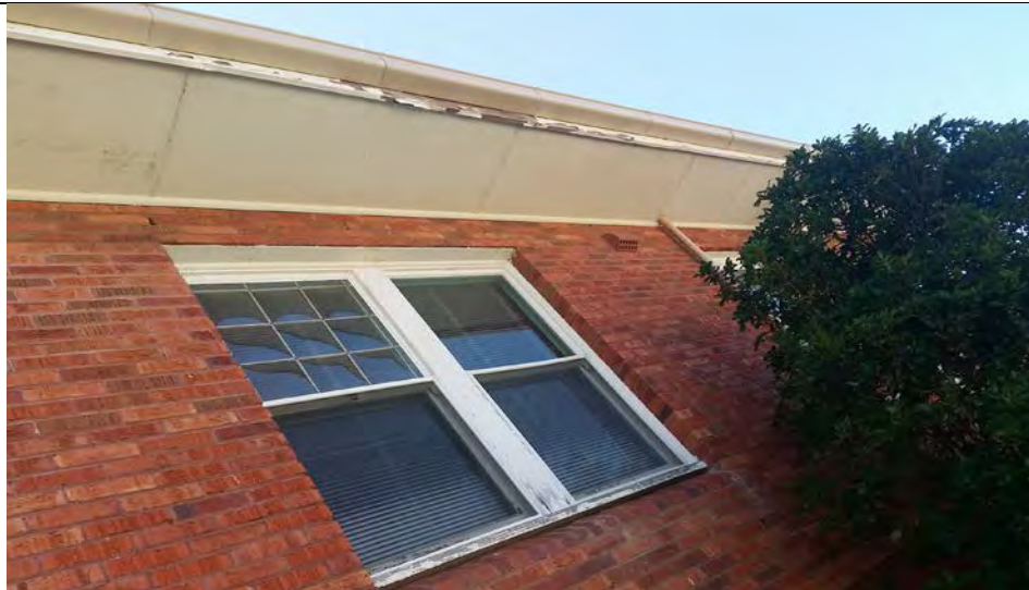
Photo 5 Building eaves with flaking paint
